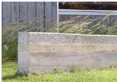
Fair-faced concrete retaining wall
